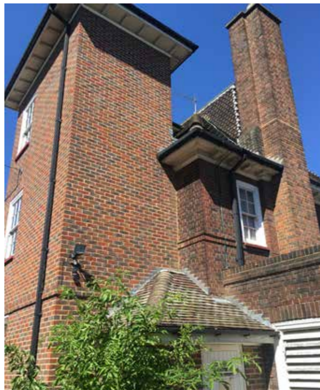
View of lift tower.
